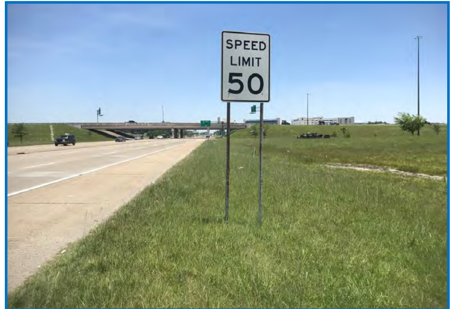
Photo 8 – View along Lloyd Expressway, facing east (6/17/2021).
