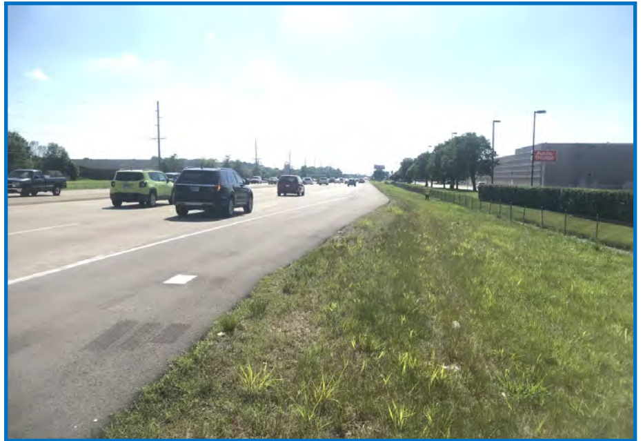
Photo 4 – View along westbound Lloyd Expressway, facing west (6/16/2021).
