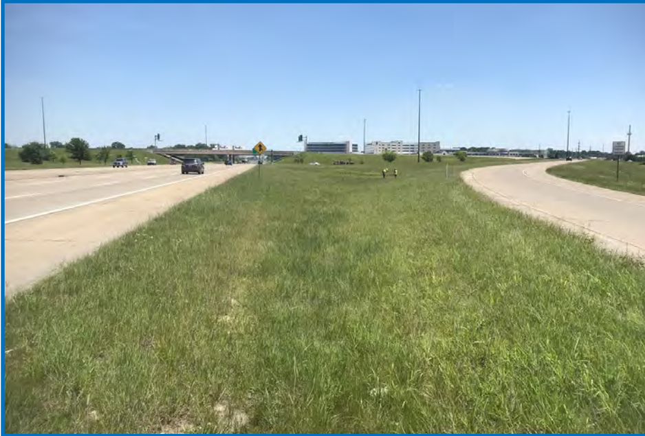
Photo 9 – View along eastbound Lloyd Expressway and the off-ramp to I-69 southbound, facing southeast (6/17/2021).
