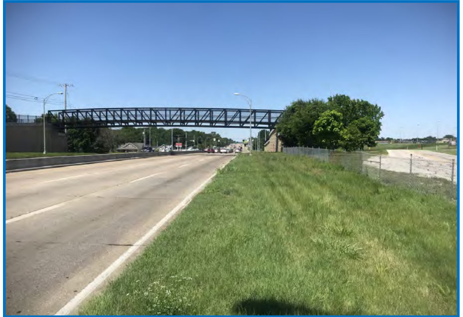
Photo 4 — View of the pedestrian bridge over Lloyd Expressway facing west (06/15/2021).
