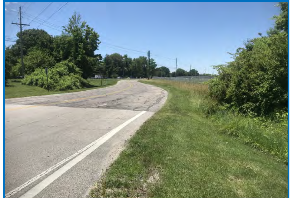
Photo 6—View of the roadside along Division Street from the Stockwell Road and Division Street intersection, facing southwest (06/15/2021).
