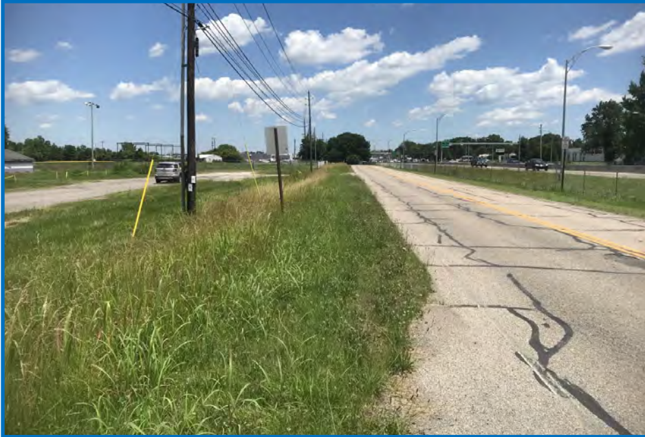
Photo 5— View of the roadside along Division Street facing east (06/15/2021).
