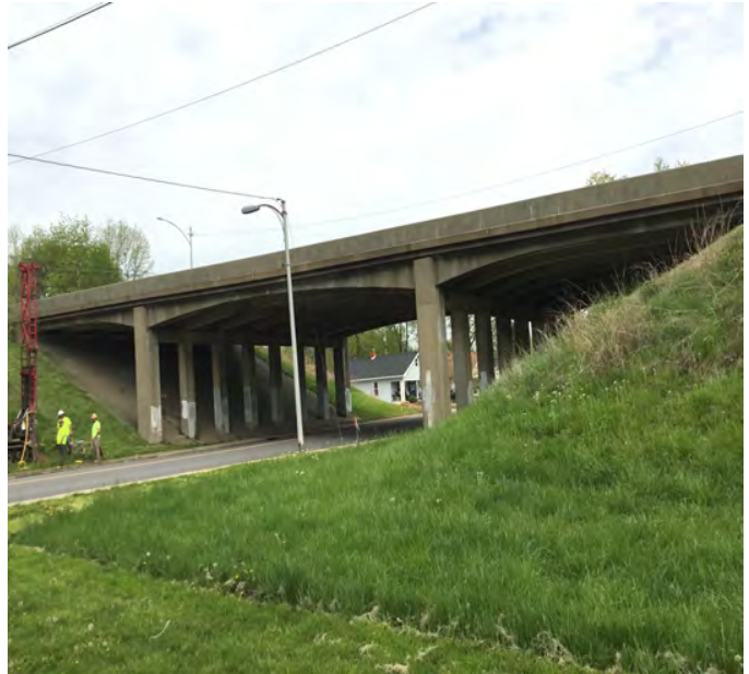
PHOTO 2 Description South Elevation.
