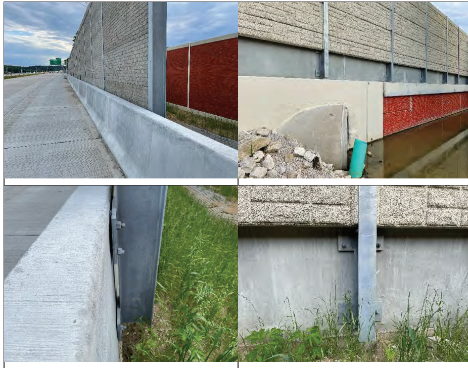
Figure 8. Noise barrier mounted to TCB on I-69 at Martinsville
