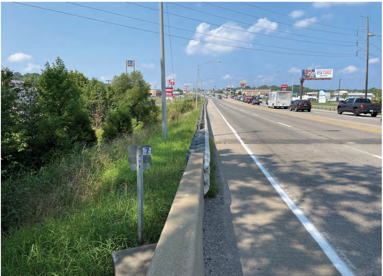
6. Facing west along south side of SR 62.
