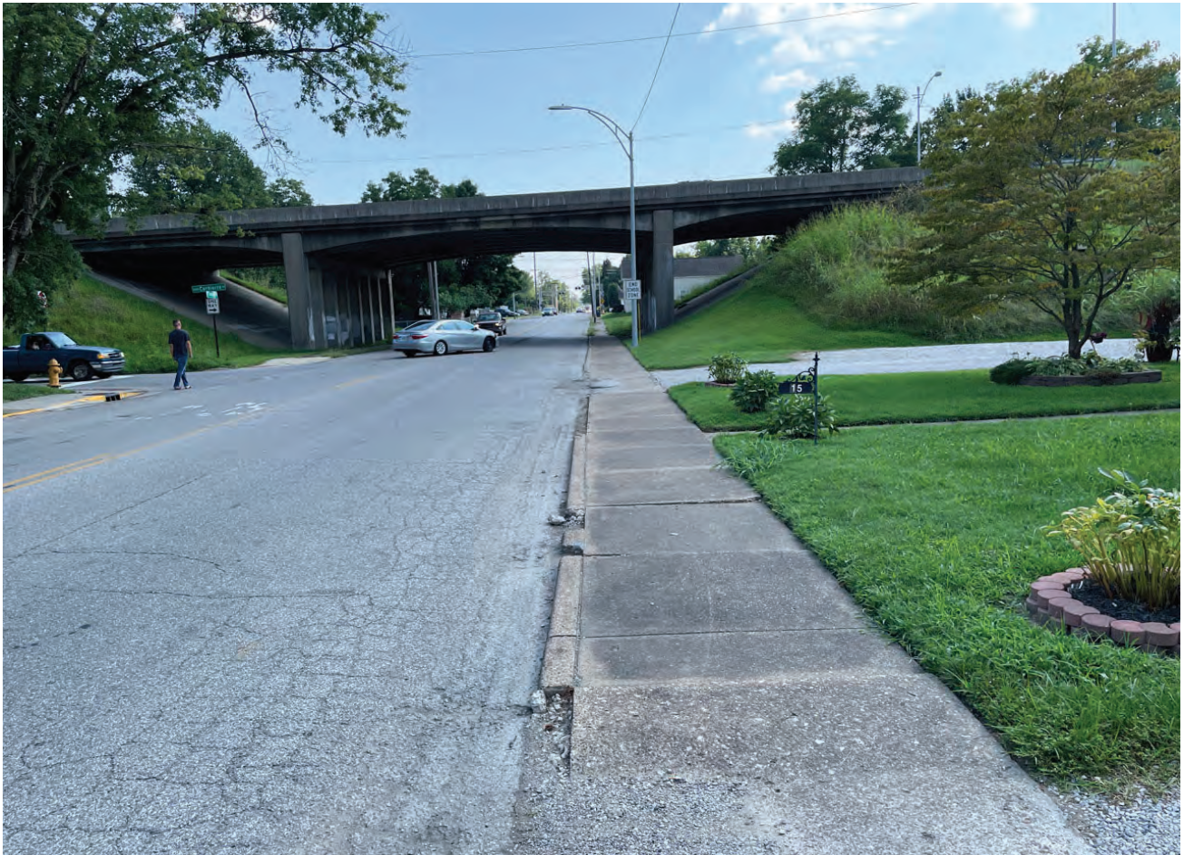
8. View of SR 62 over Tekoppel Avenue facing south.
