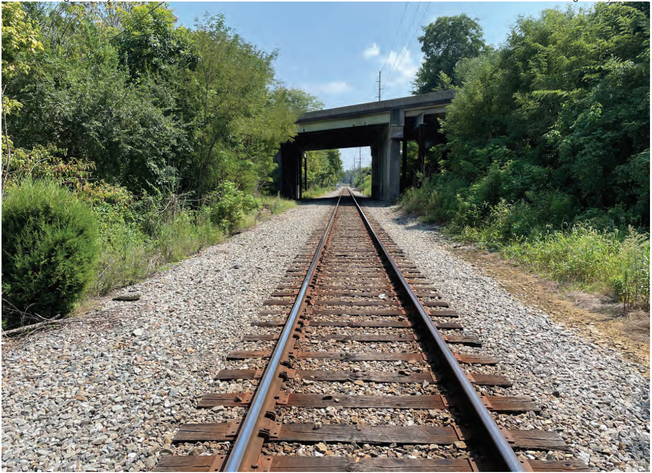
7. View of SR 62 over CSX Railroad facing northwest
