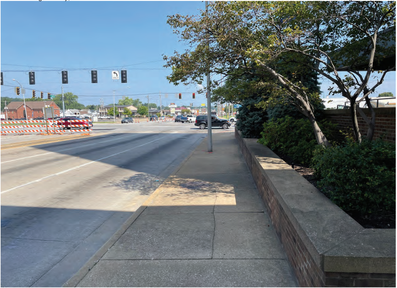
19. Facing north along St. Joseph Avenue toward SR 62 intersection, south of SR 62.
