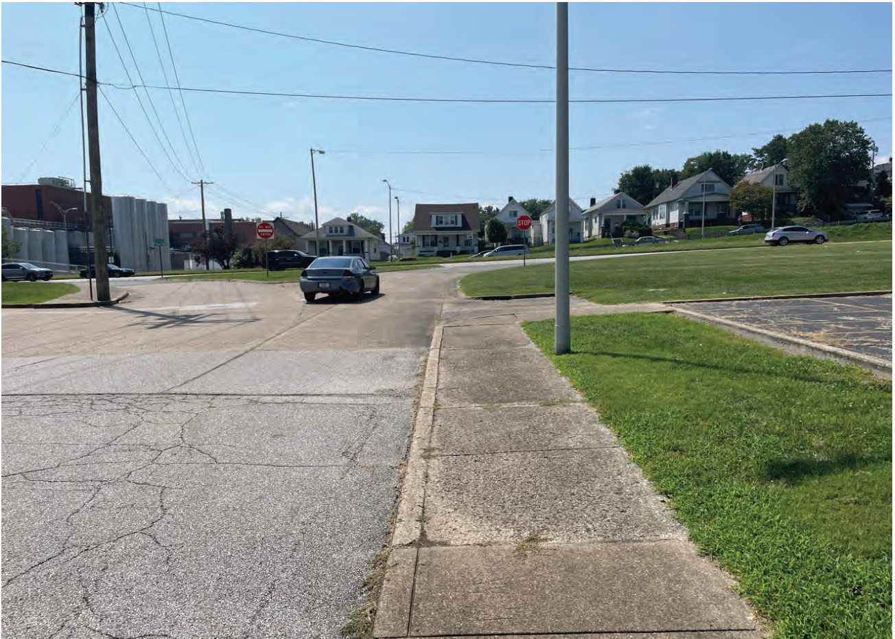
16. Facing south along Lemcke Avenue toward SR 62 intersection, north of SR 62.
